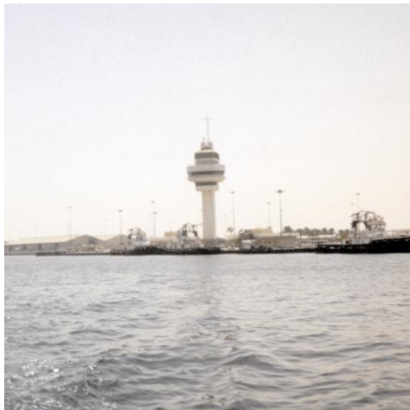
Mina Jabal Ali—Harbor Control Tower
