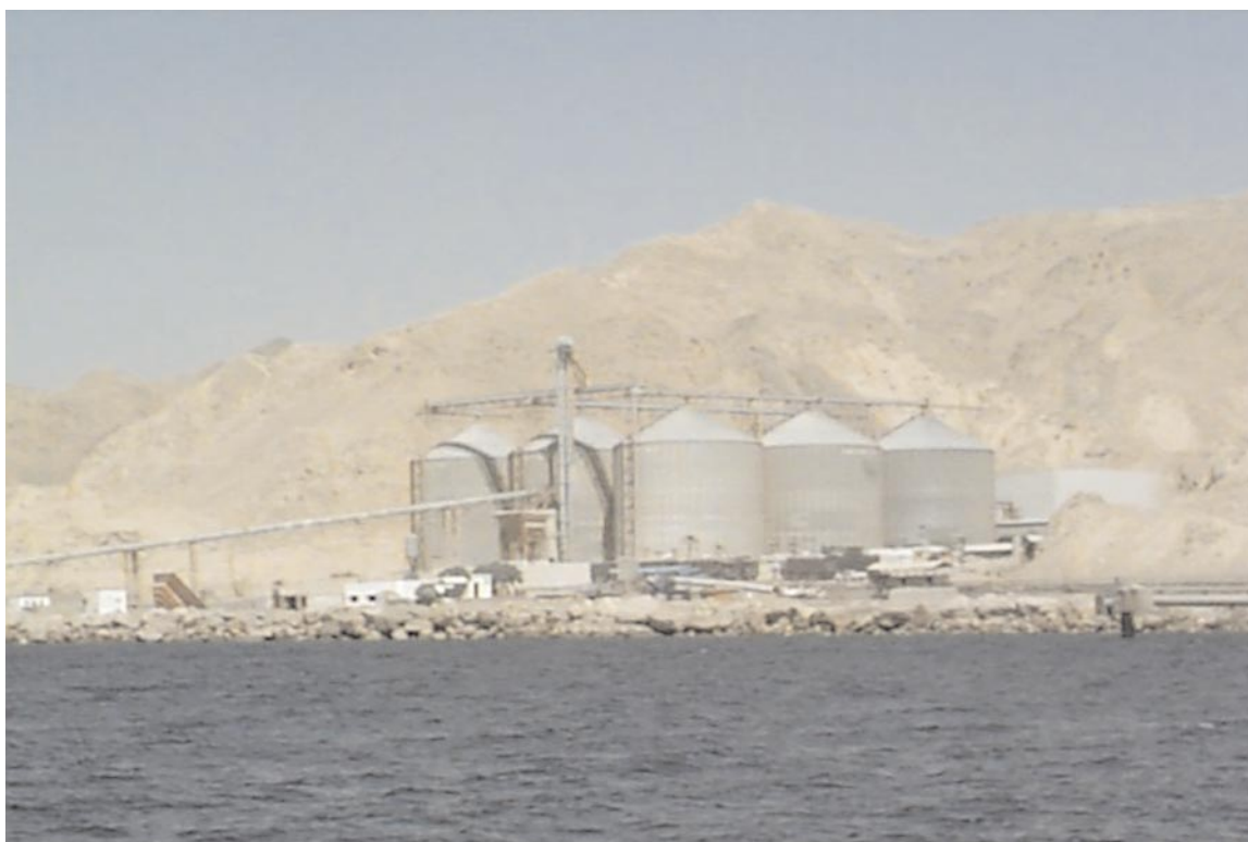
Al Aqabah—Silos close E of Mo'ta Floating Berth
