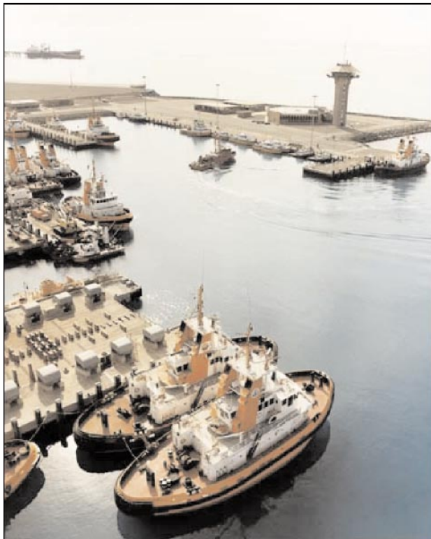
King Fahd Control Tower
