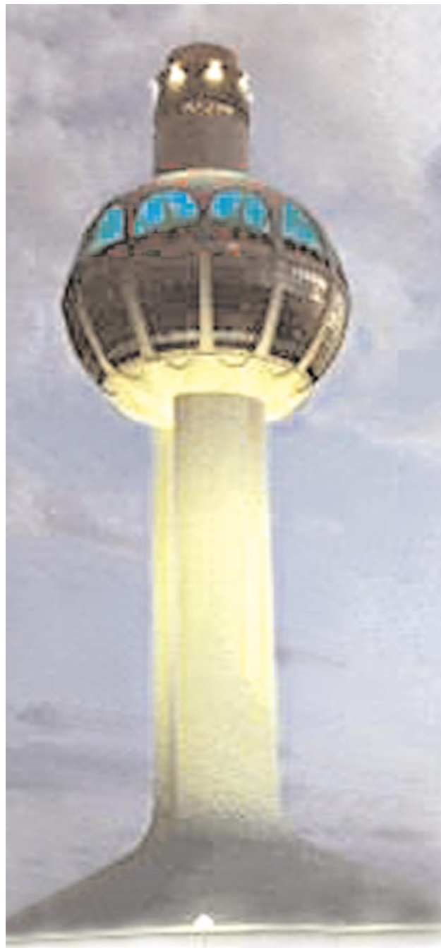
Jiddah Marine Control Tower
