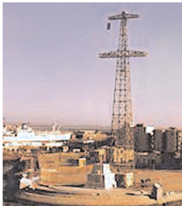
Port Suez Control Tower
