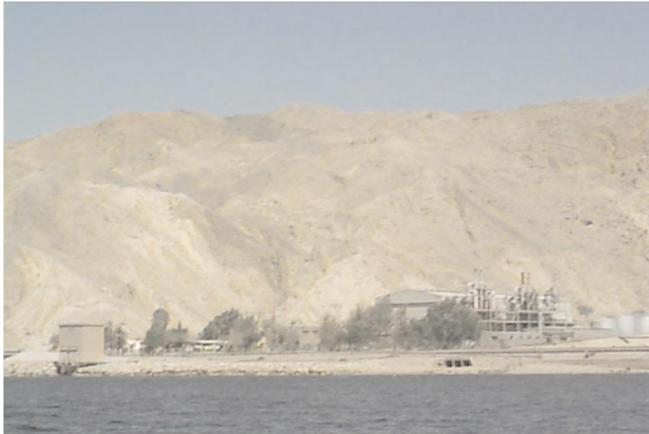
Al Aqabah—Power Station
