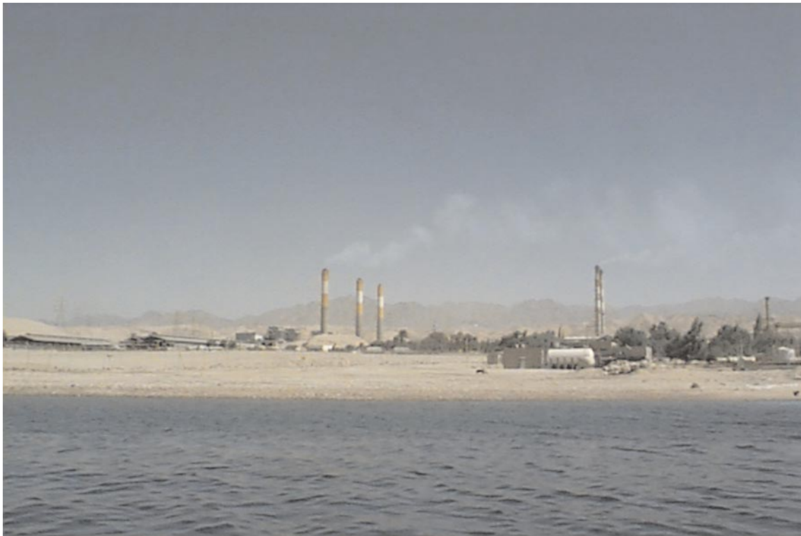
Al Aqabah—Chimneys and stacks at Jordan Fertilizer Industry facility
